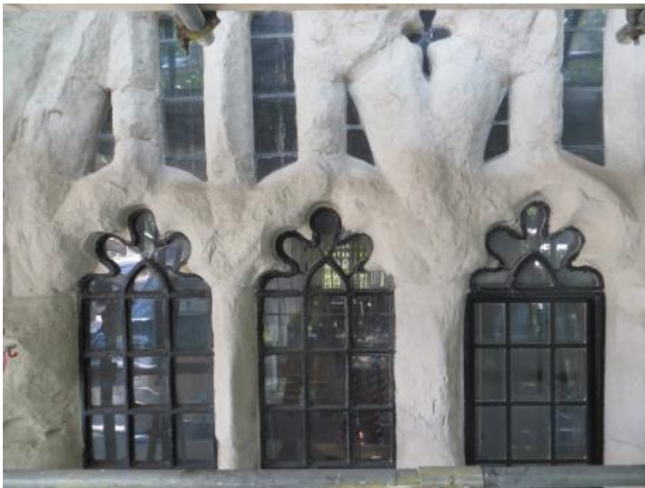
Figure 6: Repairs to window lights. Lime shelter coat applied to stone.
