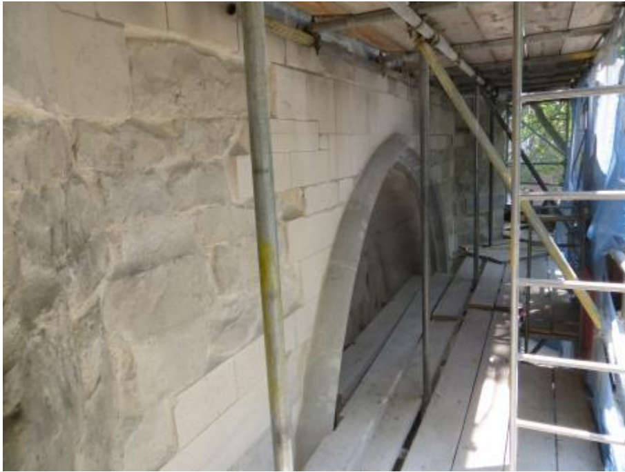
Figure 5: Replacement stone moulding over window arch
