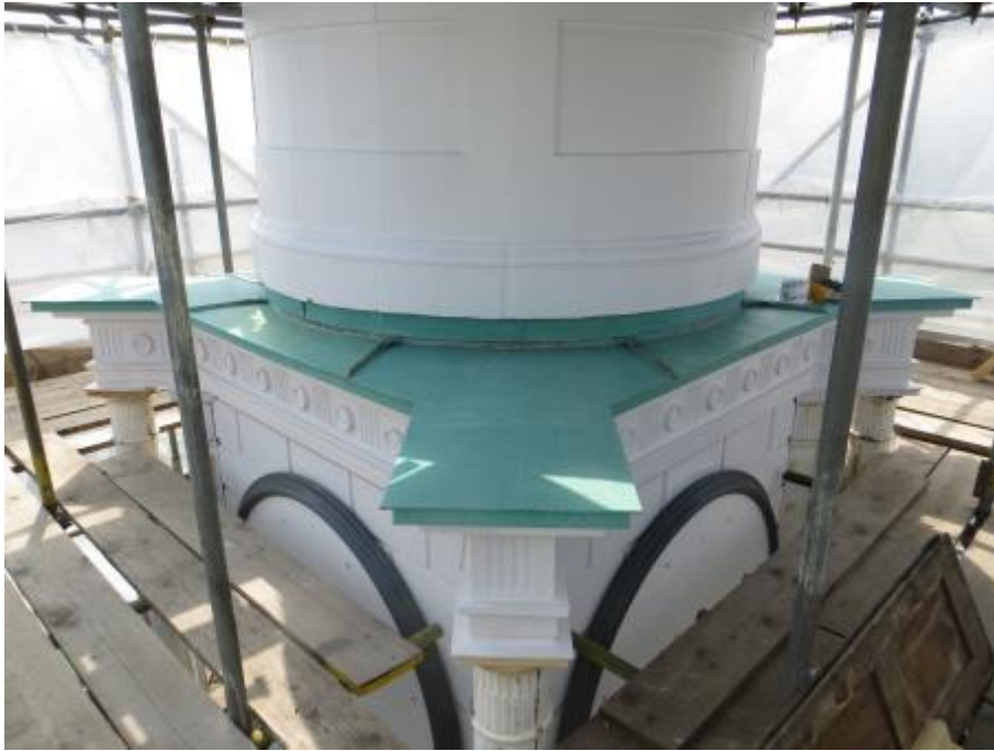
Figure 1: Bell-tower cupola replacement weather coating in weathered copper to match colour of cupola. Timber elements of bell tower repaired or replaced where necessary and painted.
